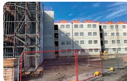
Accelerated houseblock construction, HMP Elmley
