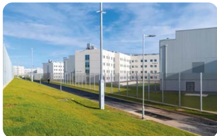
New build prison wings, HMP Five Wells
